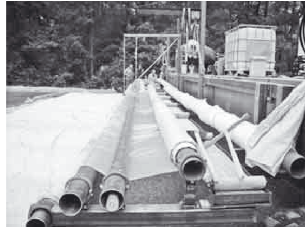
Figure 6: Working platform – device to apply foil
