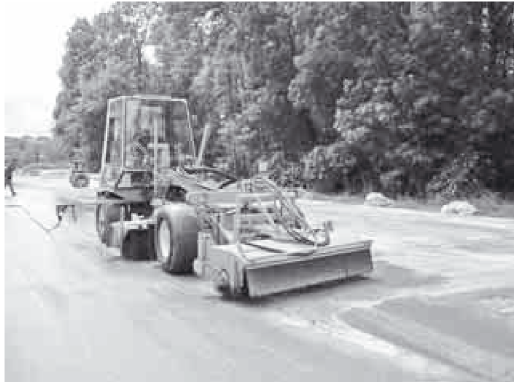
Figure 1: Brushing the surface mortar
