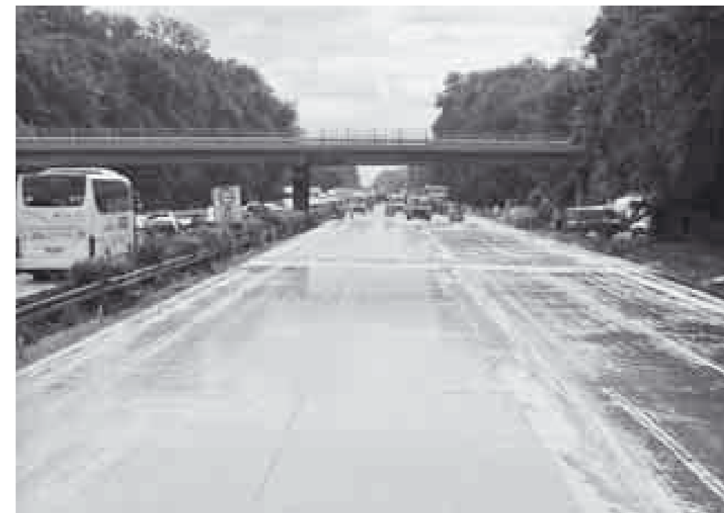
Figure 3: With foil covered concrete
