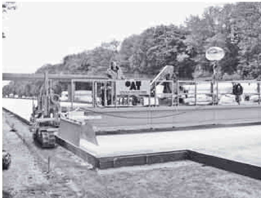
Figure 5: Working platform – spraying device
